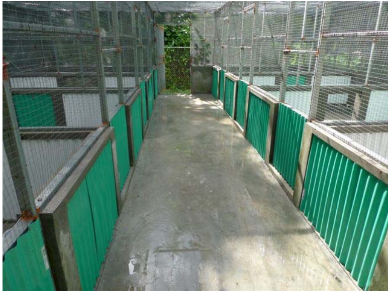
Figure 5. The final phase of the construction of the mountain chicken breeding facility on Dominica.
